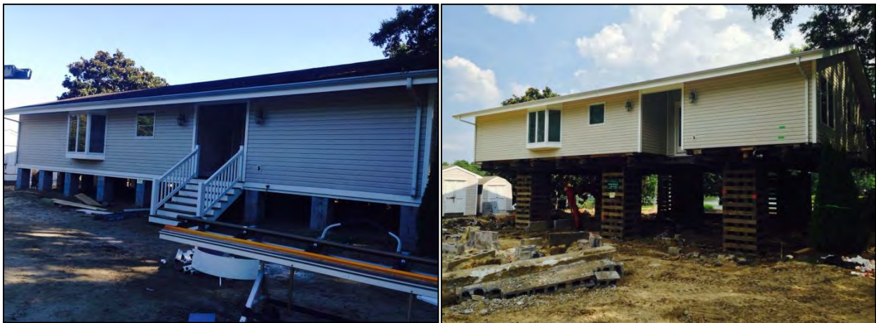
Figure 82: Photos of an elevated home in Port Haywood during (left) and after (right) being elevated (Mathews County, 2015).
