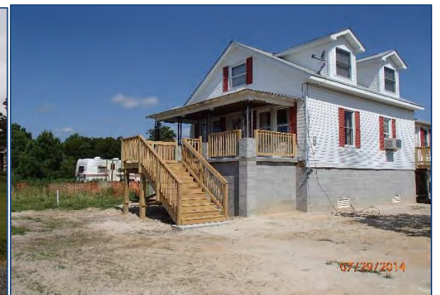
Figure 80: House in Hayes, Gloucester County - AFTER elevation.
